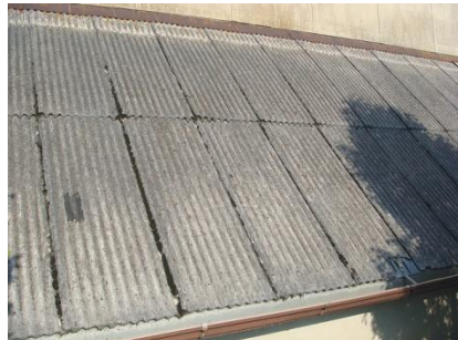
[Figure 2.c], Asbestos-cement
