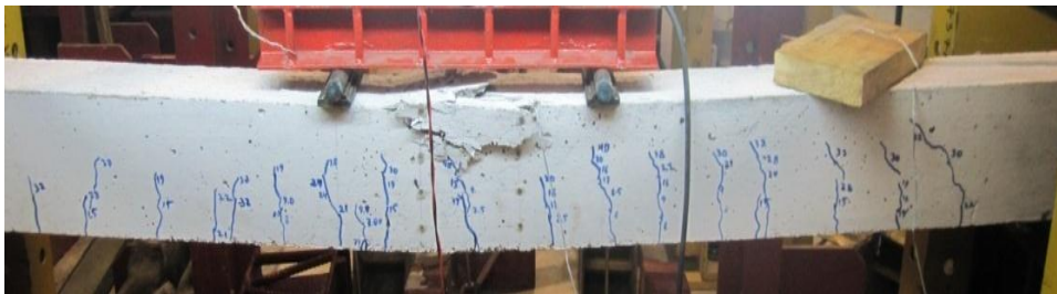
Figure 6: C30-RC beam after failure
