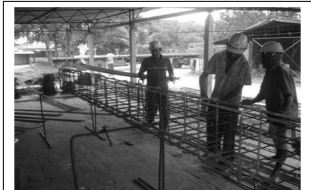
Figure 7: R/f arrangement for pre-cast tier
