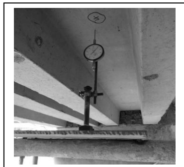
Figure 12: Dial gauges below the tiers
