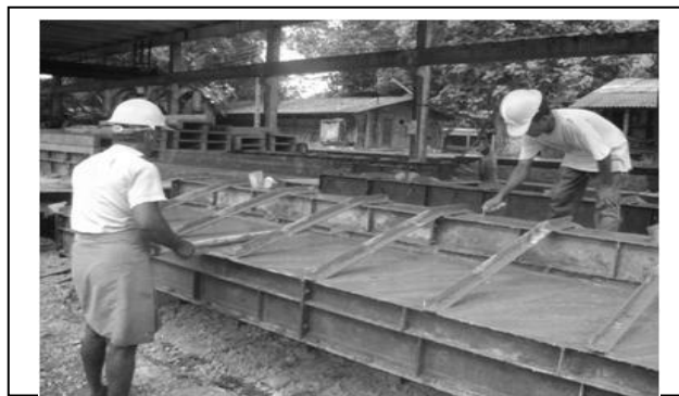
Figure 6: Formwork arrangement for pre-cast tier
