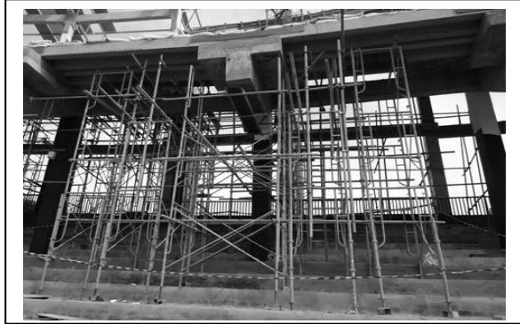
Figure 13: Loading with safety arrangement
