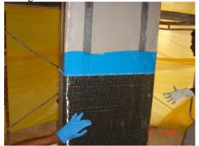
Figure 4: Application of CFRP Sheets
