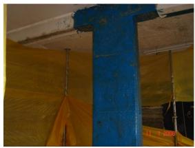
Figure 5: Finished Column before applying plaster
