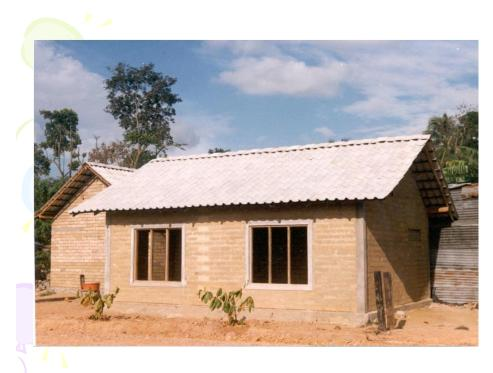
Figure 1: A house constructed with stabilized soil blocks and MCR tiles
