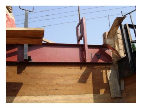
Figure 2: Rammed earth construction (A photograph taken at Center for Housing Planning and Building, Sri Lanka)
