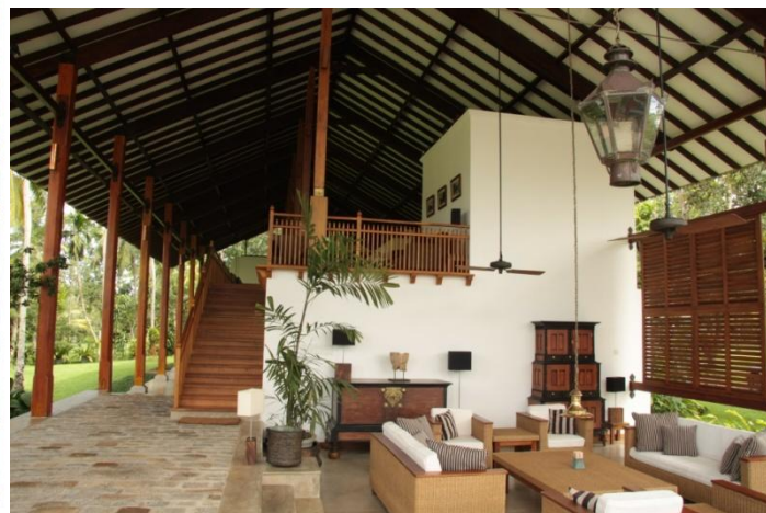
FIGURE 14 – SOLID TIMBER COLUMNS AND PORTALS
