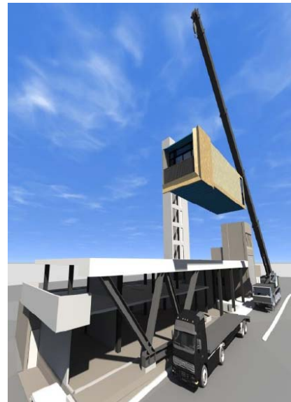
Figure 1(b): A prefabricated modular unit being brought to site for assembly
