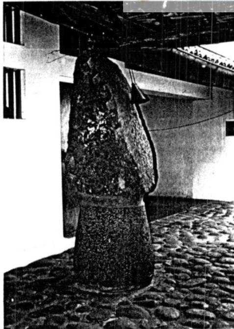
Fig.66: Roof of the entrance court, rest on a stone pillar. note: the rustic nature of materials and simple details.
