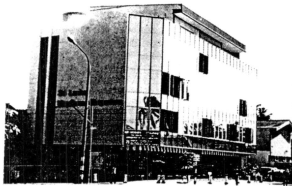
Fig. 1: Modern commercial building. Design with total disregard to local traditions.
