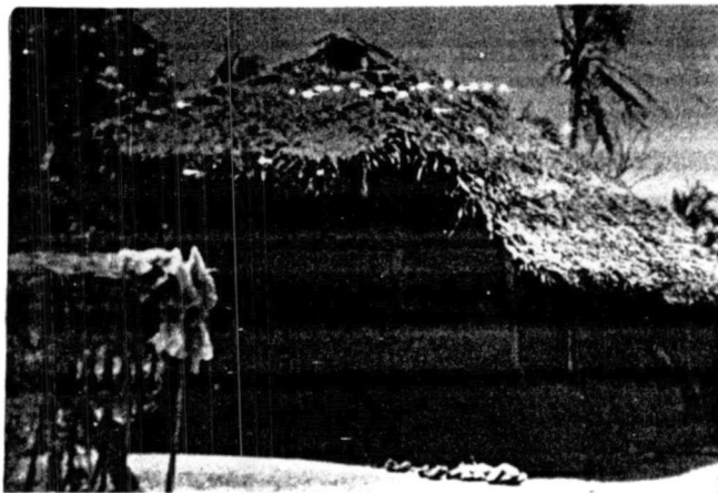
Fig.21: Peasant house – locally available materials of jungle poles and cadjan, are used for construction.
