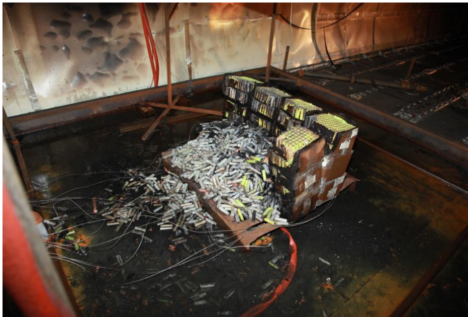
Figure 2-3: FAA fire test burnt battery load [10]
