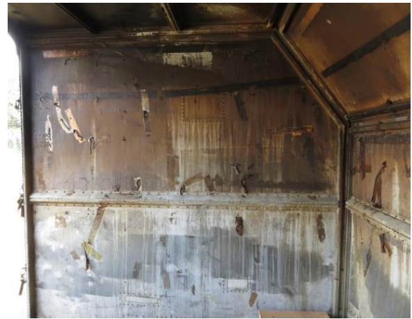
Figure 5-6: AMJ container interior fire damages
