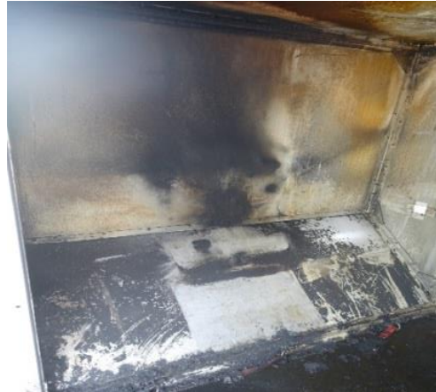
Figure 5-13: Post-test interior condition of the AKE container
