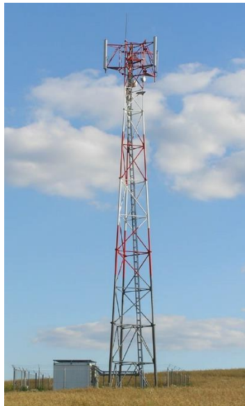
Figure 2.1 : Typical BTS with Tower and Equipment Cabin
