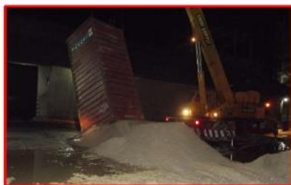
Tilting container by using cranes
