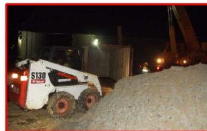
Unloading and loading container by Bobcat machine
