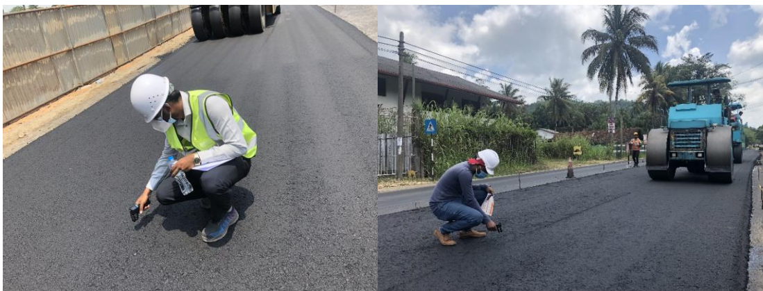
Figure 6: Measuring of asphalt surface temperature in day time
