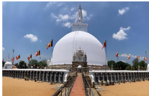
Fig. 24: 2025- Surrounding of Ruwanweliseya Source: author
