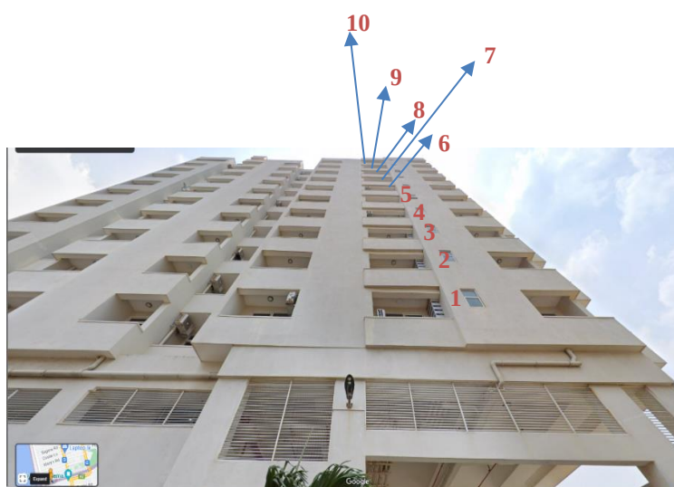
Figure 6.14: Methodology for Sample Apartment Building from the Street View and the Counting of Floors
