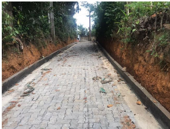
Figure 12: 12° sloped block paved road
