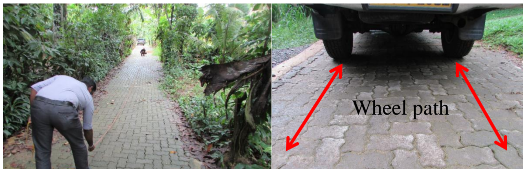
Figure 17: Identification of wheel path in completed trail road section
