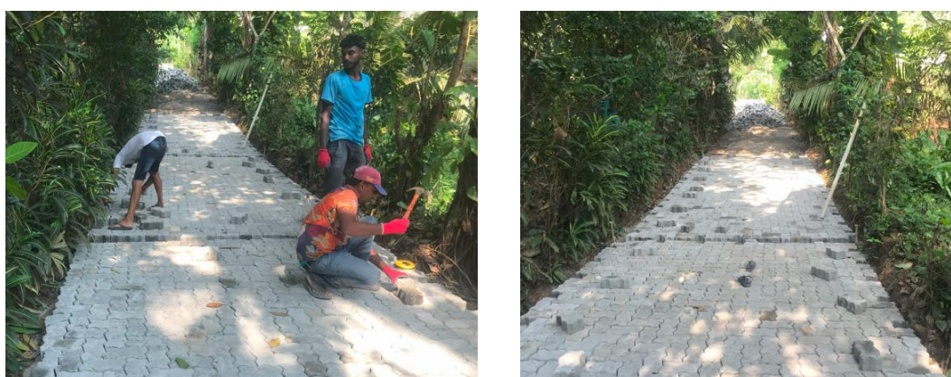
Figure 15: Block placing in trail section
