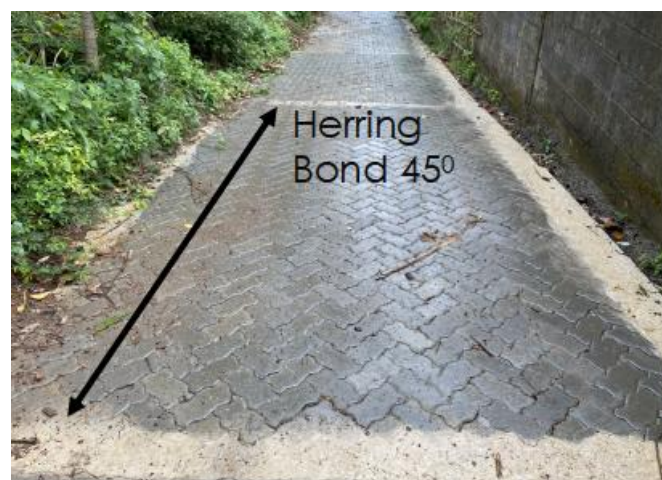
Figure 16: Finished trial block paved road section
