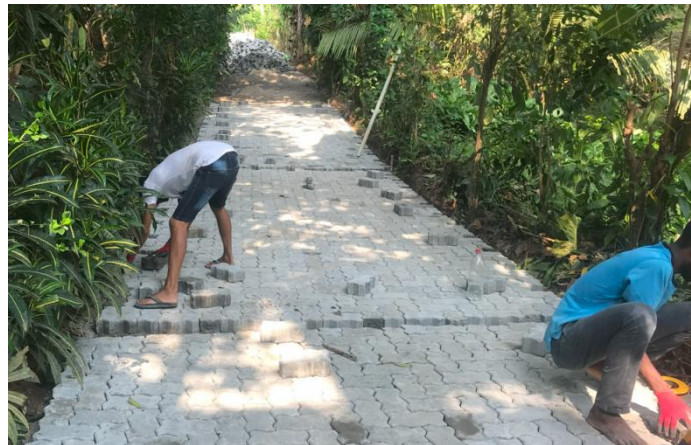
Figure 13: Common field practice of placing cross spacing
