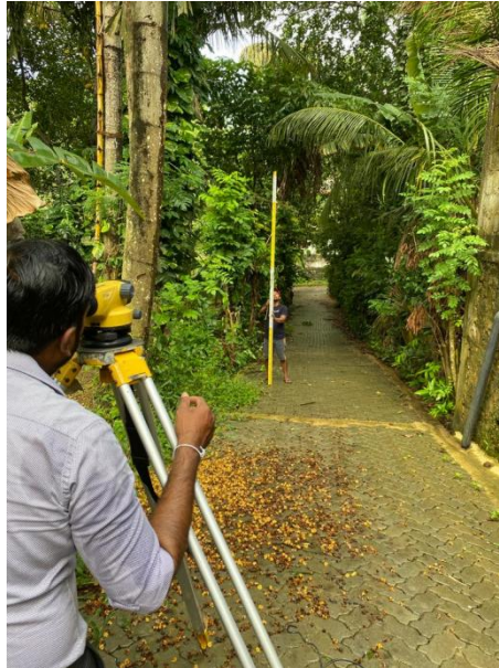
Figure 18: Surface level checking using Automatic level instrument
