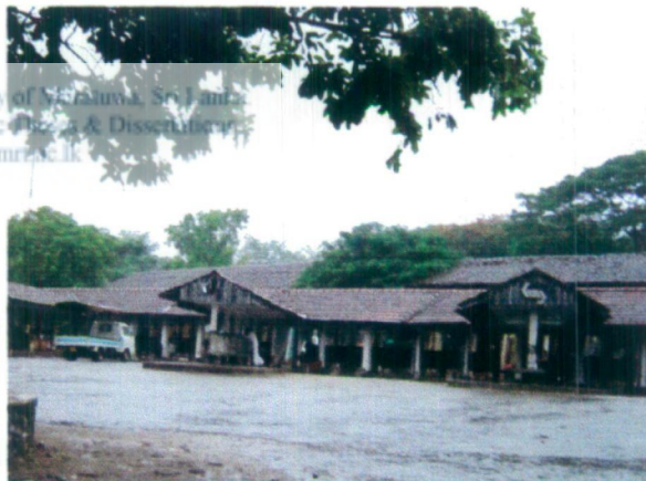
Fig. 84 - Central bus station - Girandurukotte
