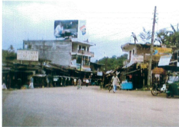
Fig. 43 - The haphazard growth of the built fabric along the Mahiyangana road Digana which has created another town centre
