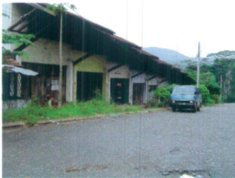
Fig. 47 - Commercial buildings Kundasale
