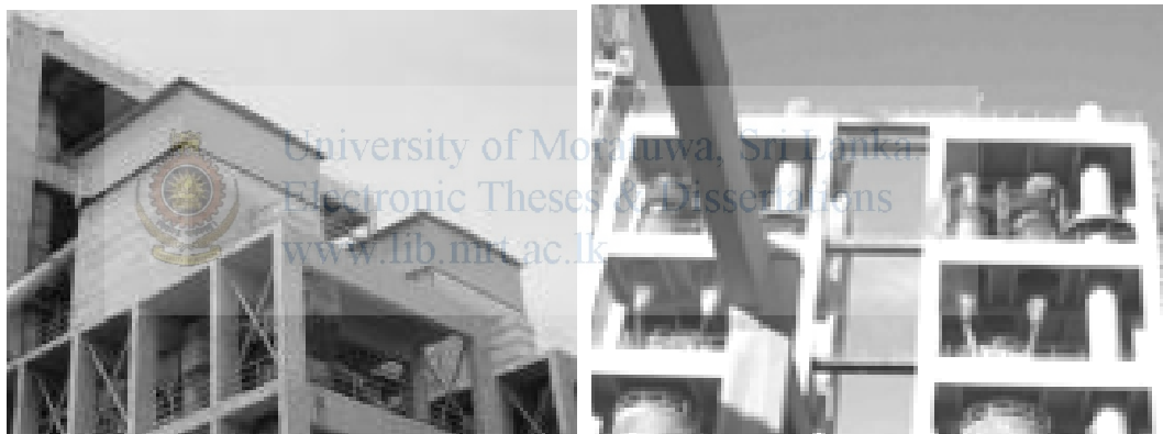
Figure 2-16: 'Blue sky' filter bag unit (L), main stacks (R) at HLL – PCW
