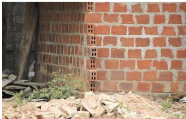
Figure 2 : Hollow Core Fired Brick (HCFB)
