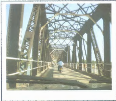
Figure 4.4 Lady Manning, Steel Bridge
