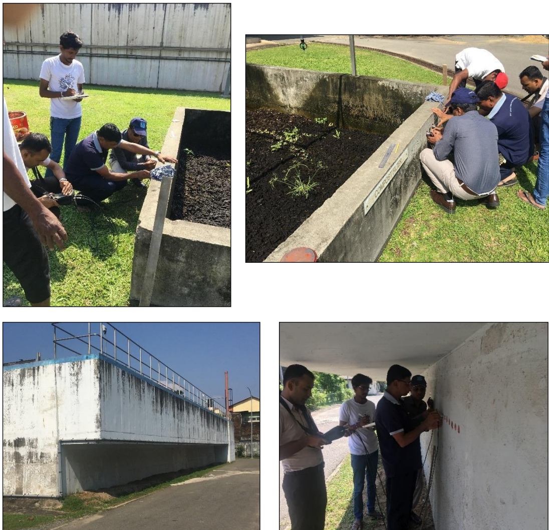
Figure 3.17; Field Measurements at Sewerage Treatment Plant, Soyzapura
