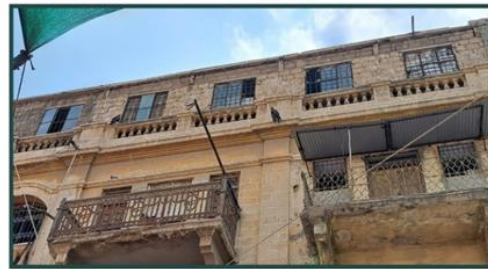
2. BALCONY, PARAPET WALL AND PILASTERS
