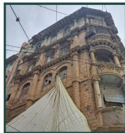
1. SIDE VIEW OF SHAMS BUILDING
