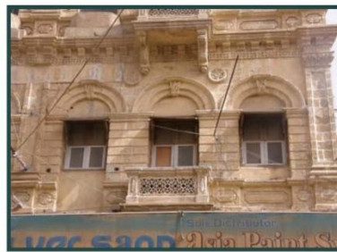
6. BALCONY, DECORATED RAILING, ROUNDELS, MOULDINGS, PILASTERS, ARCHES, KEYSTONE
