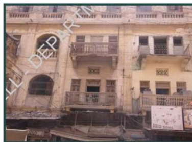
6. BALCONY, ARCHES, PILASTERS, AND BALUSTRADE
