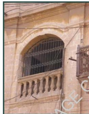
4. ARCH, PILASTER AND BALUSTRADE
