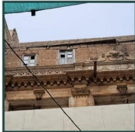
1. CORNICE, MOULDINGS, DECORATIVE PARAPET
