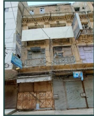
4. FRONT VIEW OF AZEEM-UDDIN BUILDING
