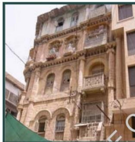
7. SIDE VIEW OF SHAMS BUILDING
