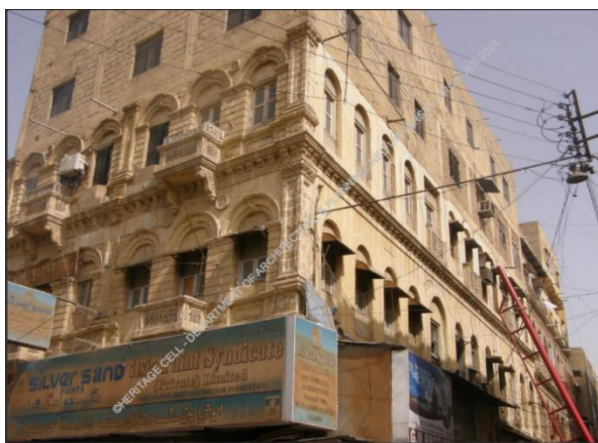
Allahwala Building, Pre 2021 Rahguzar Project Source: HC-DAPNED 2008
