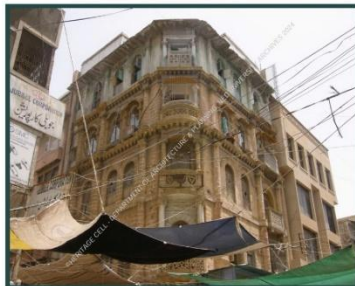
6. PERSPECTIVE VIEW OF SHAMS BUILDING SOURCE (4-5): NED UNIVERSITY HERITAGE DEPARTMENT
