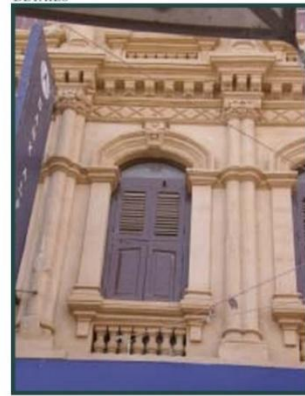
5. MOULDINGS, COLOUMN, ROUND ARCHES, KEYSTONE AND BALUSTRADE DETAILS
