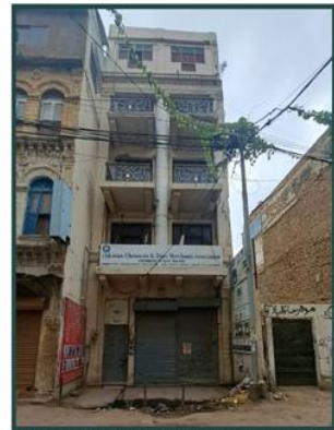
5. FRONT VIEW OF PAKISTAN CHEMICAL AND DYE HOUSE
