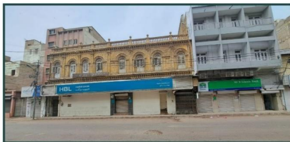
5. CONTEXTUAL VIEW OF ALVI CHAMBER
