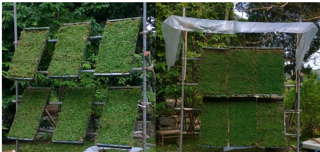
Figure 6.9: Setting up the modular panel green wall system
