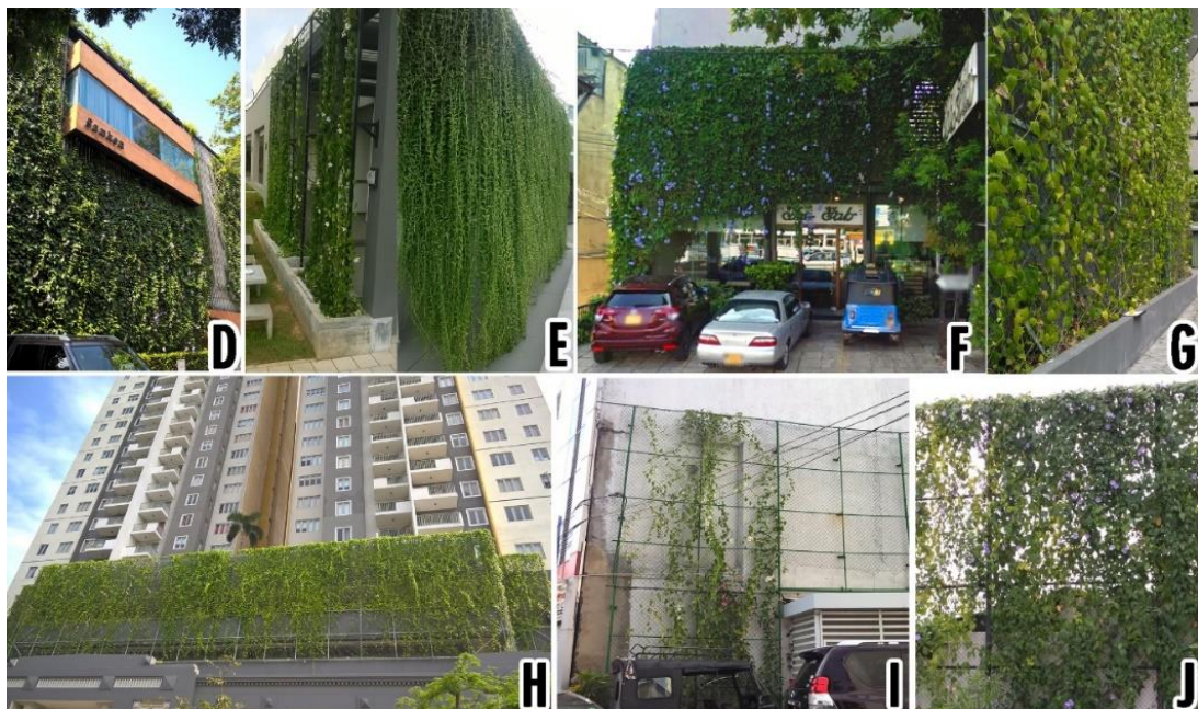
Figure 4.3: Indirect green facades in Colombo context
