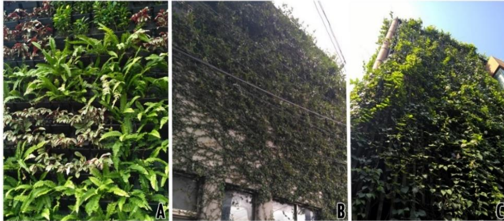
Figure 4.19: Selected case studies for further on-site investigation (A- Living wall, B- Direct green façade, C- Indirect green façade)
