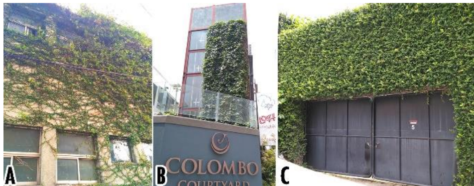
Figure 4.2: Direct green facades in Colombo context
