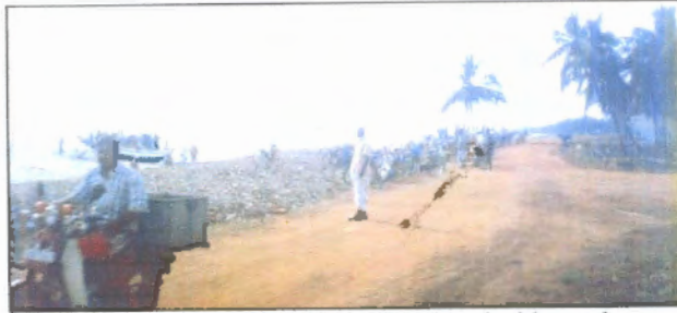
Fig 4.3 Reconstruction of the beach side road
