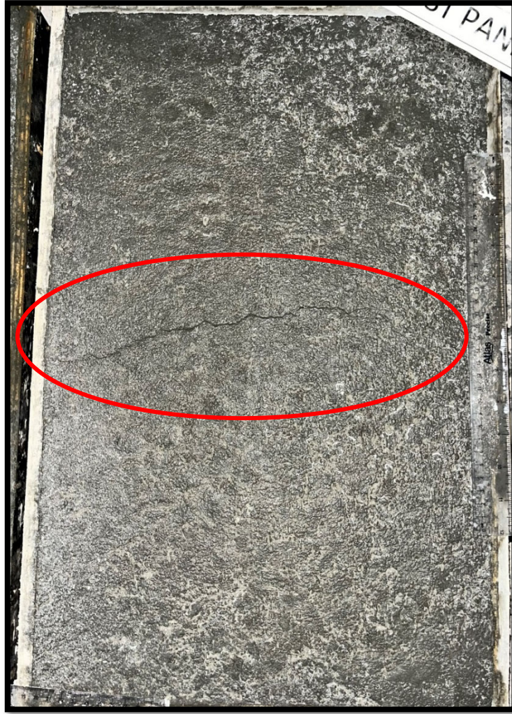
Figure 4.12 : Crack pattern of the concrete mix of fresh concrete temp. 36.0 °C
