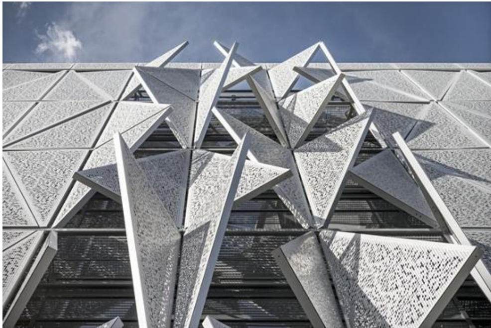
Figure 41: Shutters on the Kolding Campus (image courtesy of Jens Lindhe) [42]
