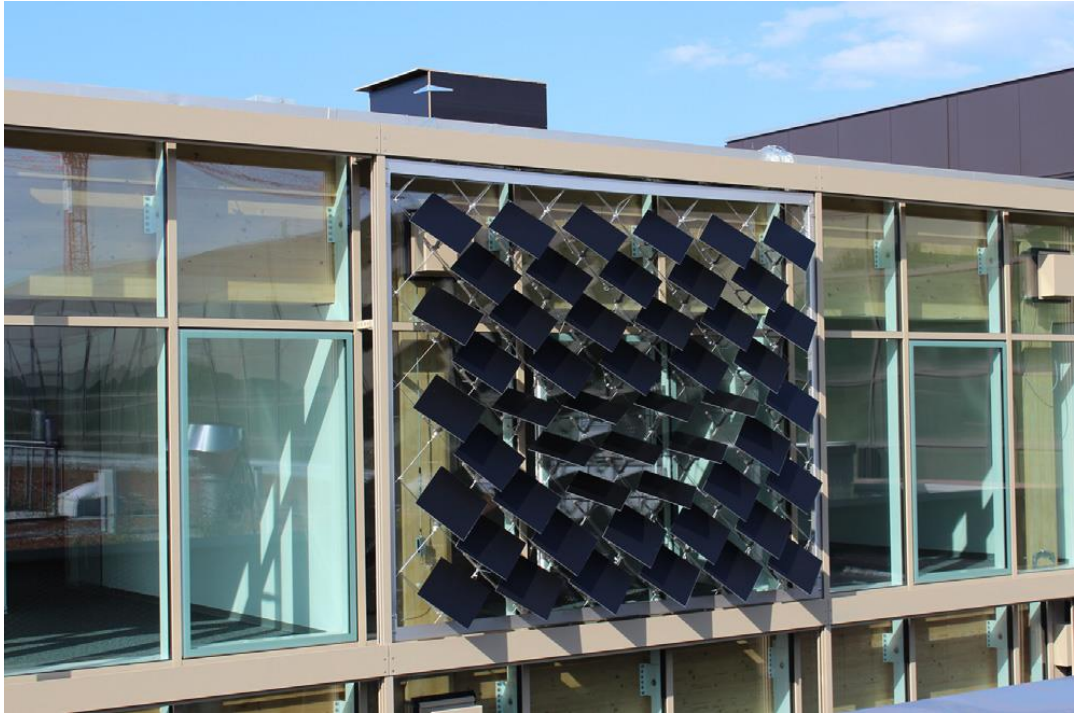
Figure 34: Adaptive Solar Façade [38]
