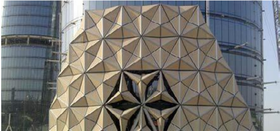
Figure 6: Al Bahar Towers in Abu Dhabi - adaptive shading façades [26].
