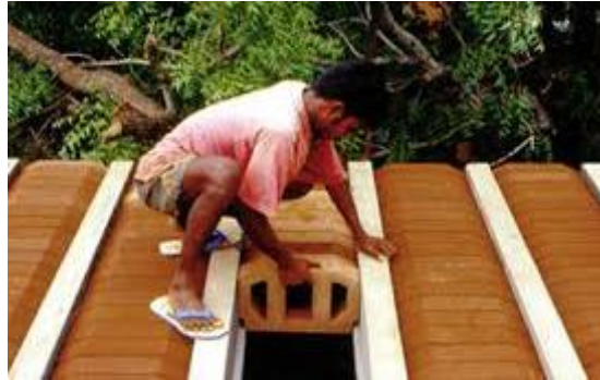
Figure 3: Image showing construction of Hourdi roof. Source: (Auroville Earth Institute, n.d.)
