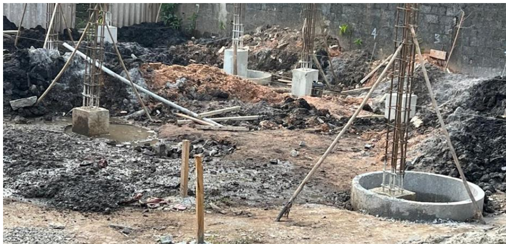
Figure 1-4: Cylinders filled with quarry dust
