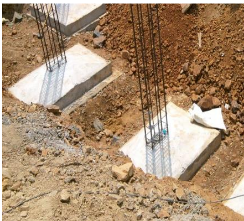
Figure 1-1: Individual Pad Footing
