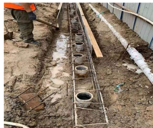
Figure 2-2: Micro pile group
