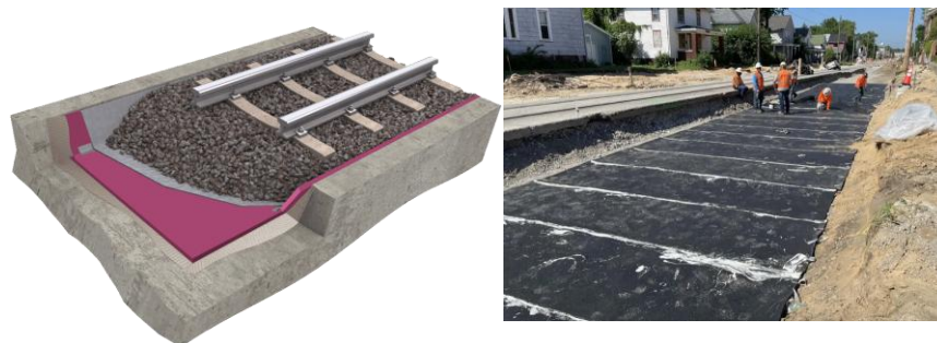
Figure 2.17: Illustration of BM and its installation
