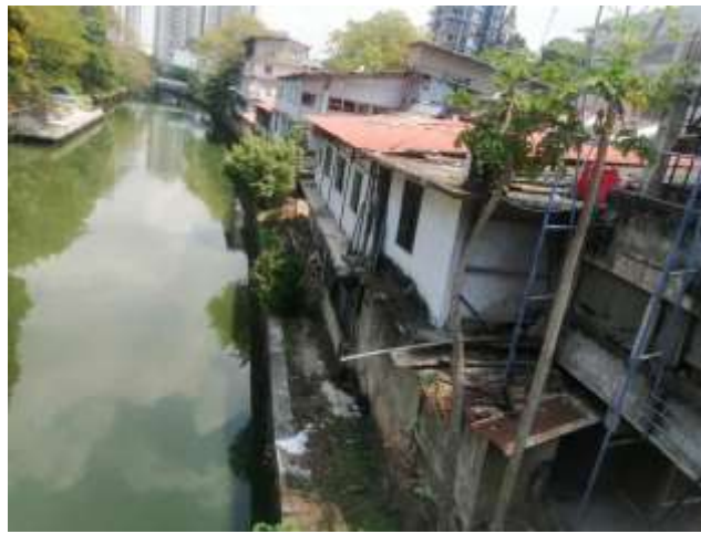
Figure 2.35: Project site as seen today after the remediation sheet piles
