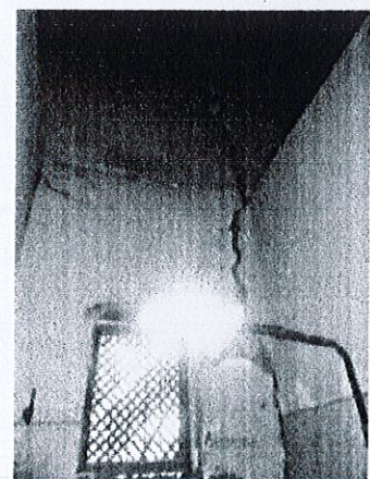
Fig. B.6 Cracks in walls at single story area (at rear and by the side of two story portion).
