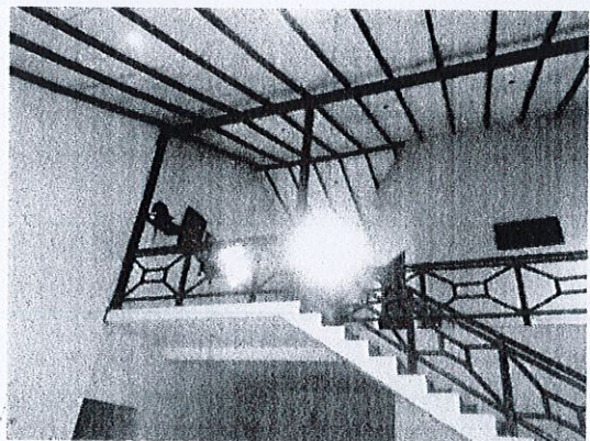
Fig. B.5 Cracks in front varandha columns and arrangement of roof rafters, some of which are about to dislodge from their connections
