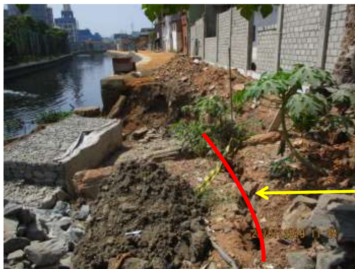
Figure 3.5: Ground movement at the back side of the House Ref No. P61.
