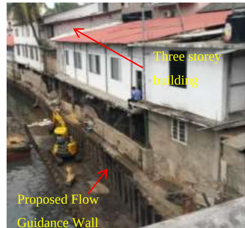
b) Building during construction stage
