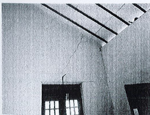
Fig. B.3 Wall and floor cracks in single storied front (living) area
