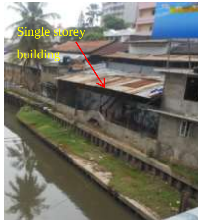
a) Building during design stage
