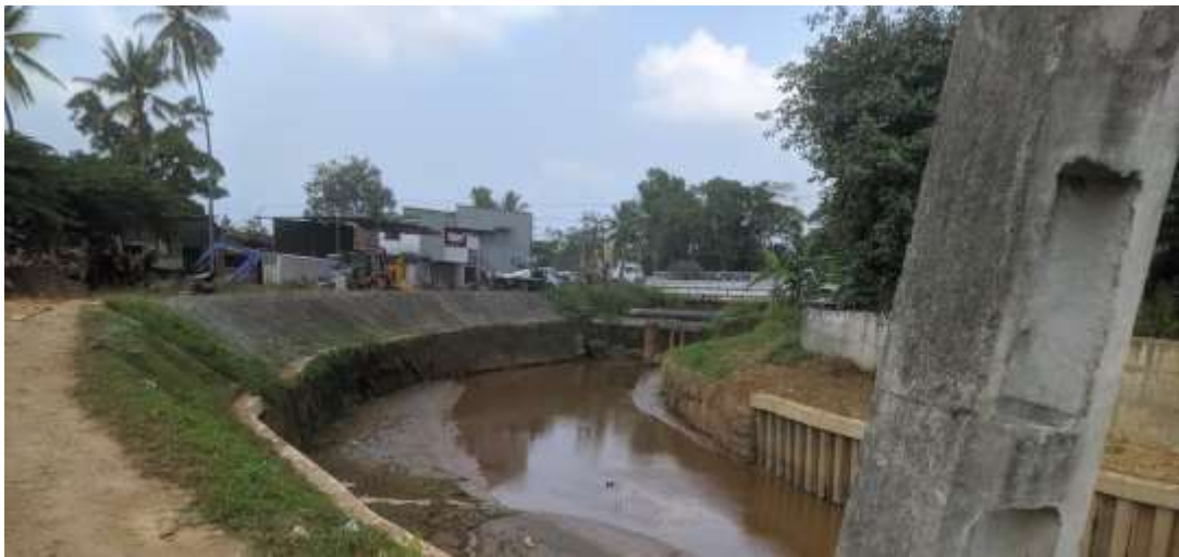
Figure 2.12: Completed canal bank protection as seen now.
