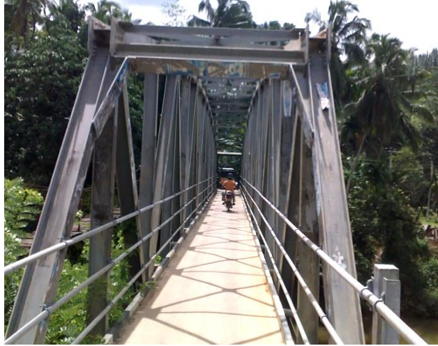
Figure 3.3: Variable height Gangasiriya Bridge
