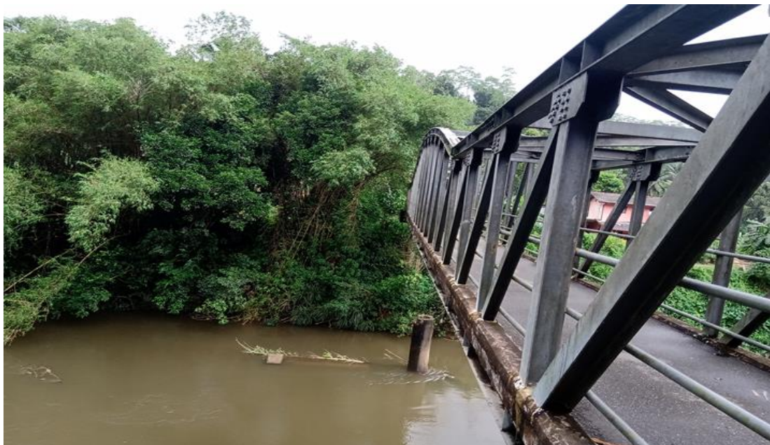
Figure 3.13: Parts of the old bridge under existing Ehalakanda Bridge
