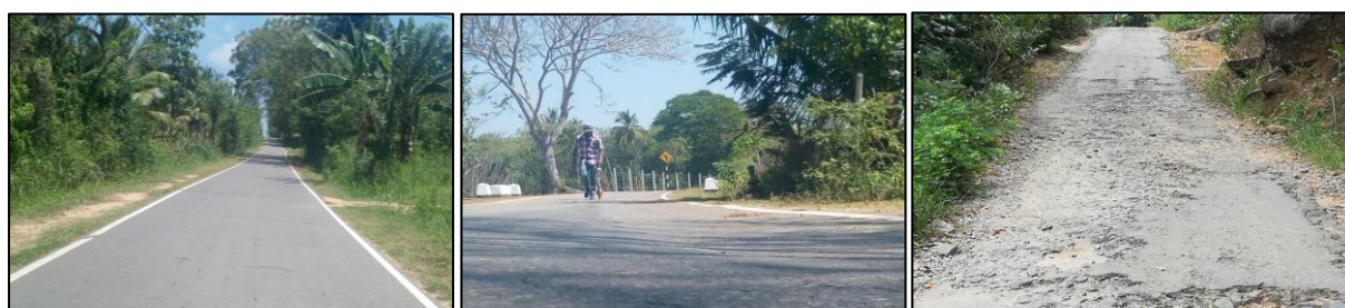
Figure 3-1: Example of Road Sections with Different Distress Levels in The Low Volume Rural Road Network
