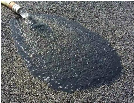
Figure 2: Porous Asphalt Pavement
