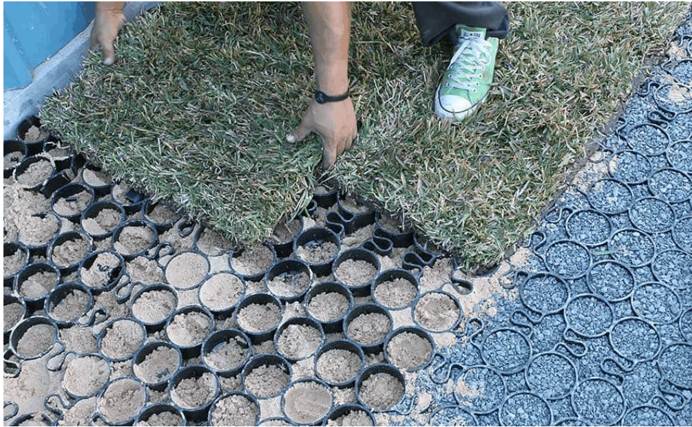
Figure 6: Plastic Grid Pavement filled with grass and gravel
