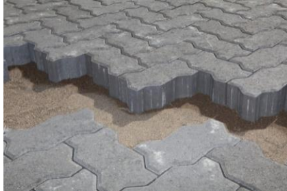
Figure 4: Permeable interlocking concrete pavement
