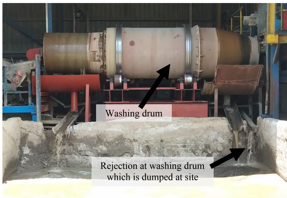
Figure 15: Washing drum of the recycling plant
