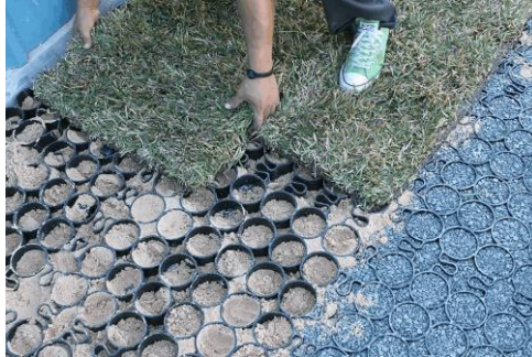
Figure 3: Plastic Grid Pavement filled with grass and gravel
