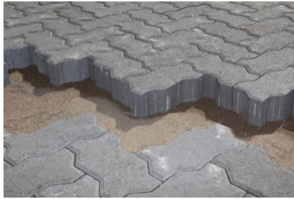
Figure 1: Permeable interlocking concrete pavement
