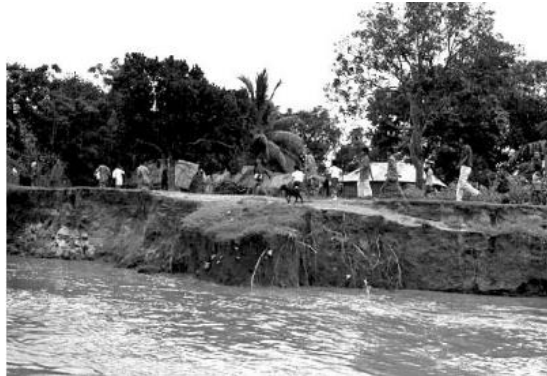
Figure 2.2 Failure of River Bank
