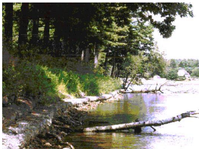
Figure 2.17 showing the post-construction performance
