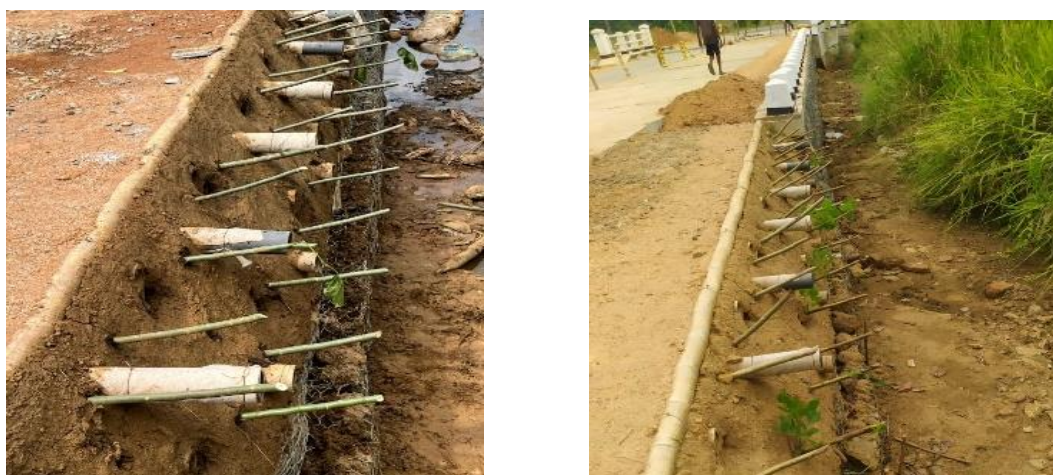
Figure 3.22 Photographs taken at Location 2 on 21.03.2024 after the stabilization technique
