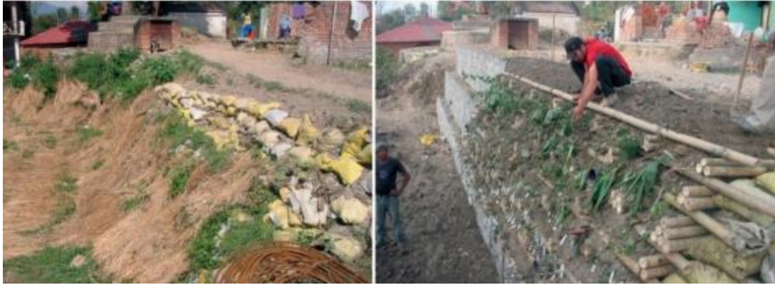
Figure 2.18: Kusunti, Lalitpur, before and after construction photos
