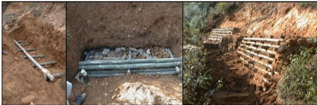
Figure 2.9 Stages of bamboo crib wall construction
