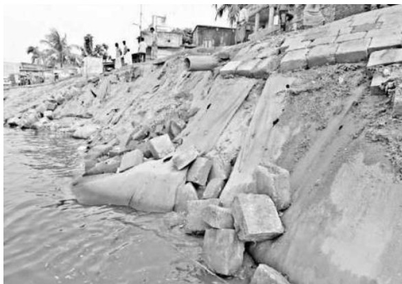
Figure 2.15 The Keraniganj Beribadh site's CC blocks are performing poorly
