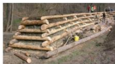
Figure 2.7 A wooden crib wall example
