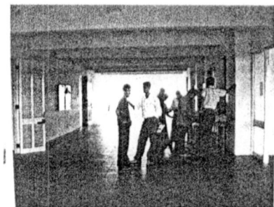
Fig 4.2.6: The lobby at Ground level –Auditorium building
