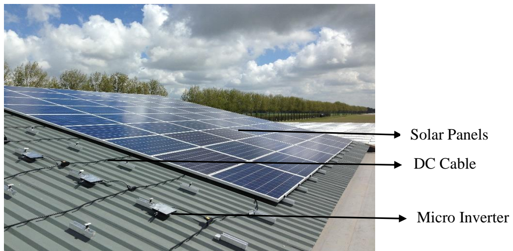
Figure 2.18: Installation of Micro Inverters on a roof
