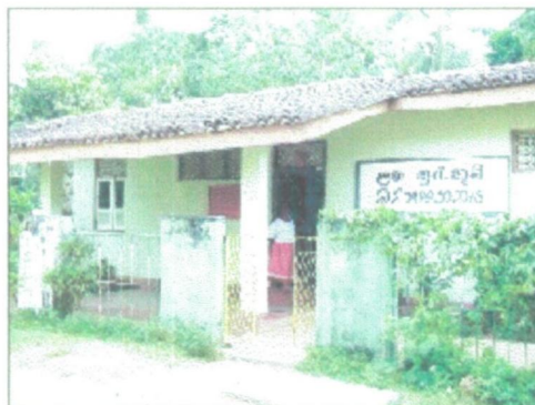
Figure 36- A day care center has been built by the occupants’ welfare society
