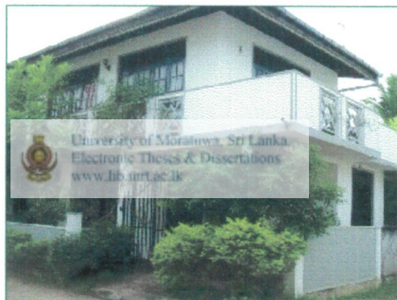
Figure 57- People expect less privacy have built low boundary walls and large balconies.
