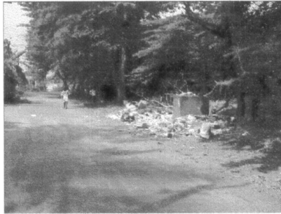
Figure 75- undesignated areas have maintenance problem.
