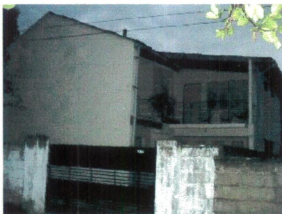
Figure 40- High boundary walls have been built to high security.
