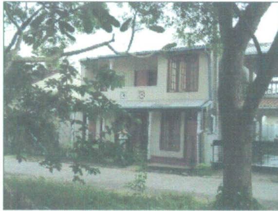
Figure 41- Large openings and balconies were added to increase the possibility of seeing alternative views from their house and to improve the cross ventilation. ( Type “D”)
