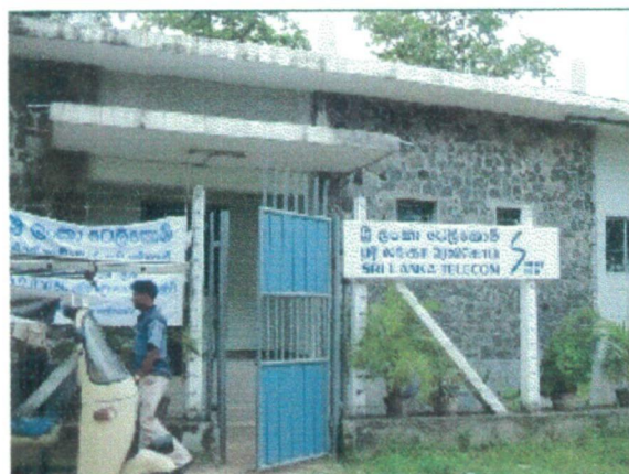
Figure 17- Telecom substation to provide the telephone facility.
