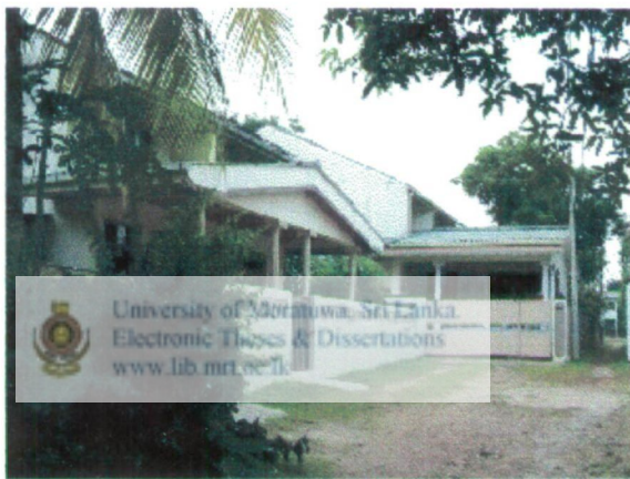
Figure 50- Different roof structures have been used with different colours.
