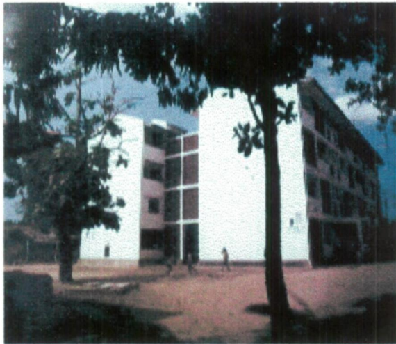
Figure 11- Sameness in four storied flats.
