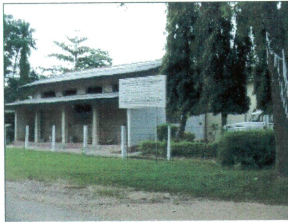
Figure 15 - Water treatment plant in the located in the scheme
