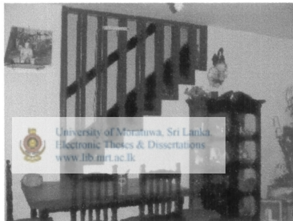
Figure 81- The stair case has been modified with a decorative timber slats by removing the existing wall to gain variety.
