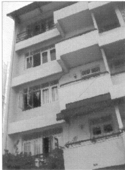
Figure 102- The modification, which has been done to gain livability is help to give identity to the topmost level house.
