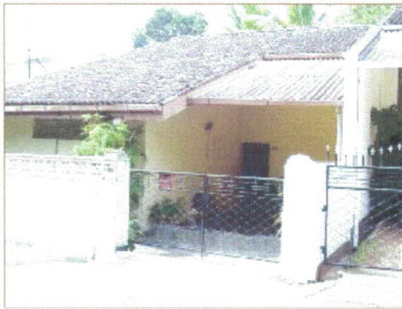
Figure 91-A roof has been extended to expand the front verandah due to insufficient space of type “C”
