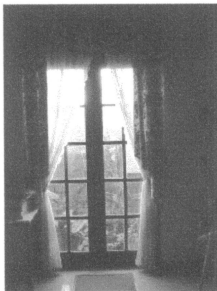
Figure 76- French windows have been used to improve the cross ventilation and seeing alternative views from their house. ( Type “A”)
