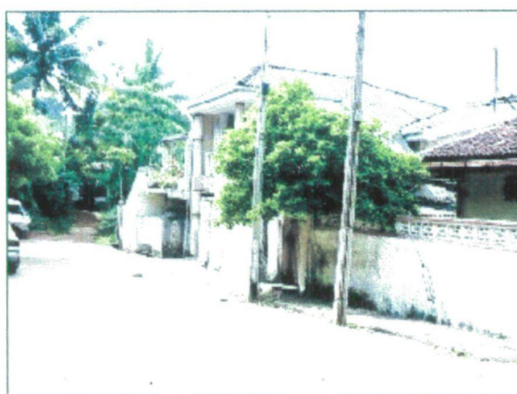
Figure 84- Different roof structures have been used to identify separately from others. ( Type “E”)
