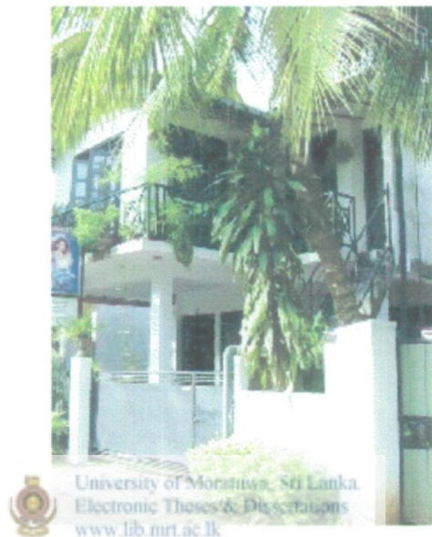
Figure 48- Two bed rooms have been added by modifying a “D” type house
