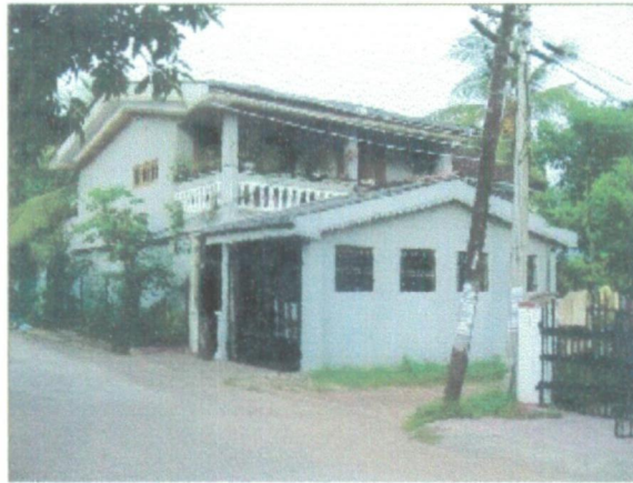
Figure 62- Enclosure has been expanded by adding a poach.
