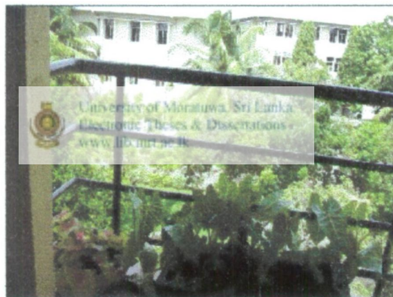
Figure 98- Houses were modified with steel frames to improve the degree of getting cross ventilation and see alternative views.
