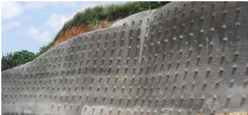
Figure 4-6. Shotcrete facings with strengthened nailhead area
