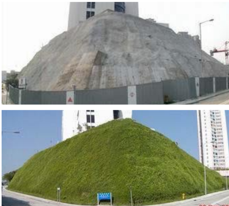
Figure 8-1. Vegetation cover on steep shotcrete slope (before and after)
