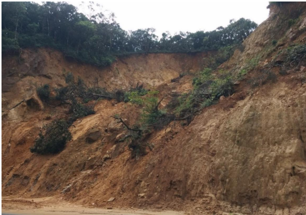
Figure 3-2. Image of Hakgala major landslide before implementing mitigations
