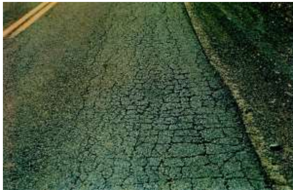
Figure 3.11: Fatigue cracking in flexible pavements
