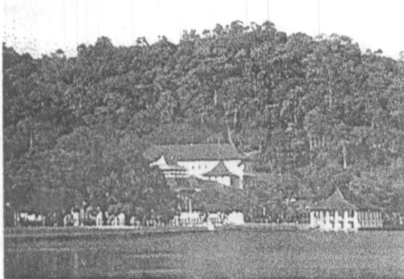
Fig. 4.0.4 The Temple of Tooth Relic in Kandy; The last link of the Sri Lankan Traditional Architecture.
