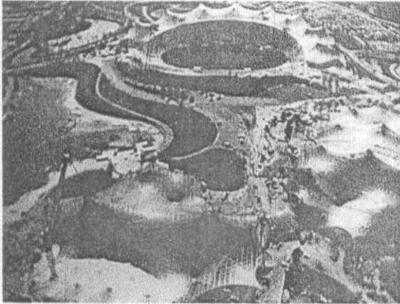
Fig. 3.5.9 Tent roof structure blend with the surrounding Mountains, Olympiastadion in Munich.
