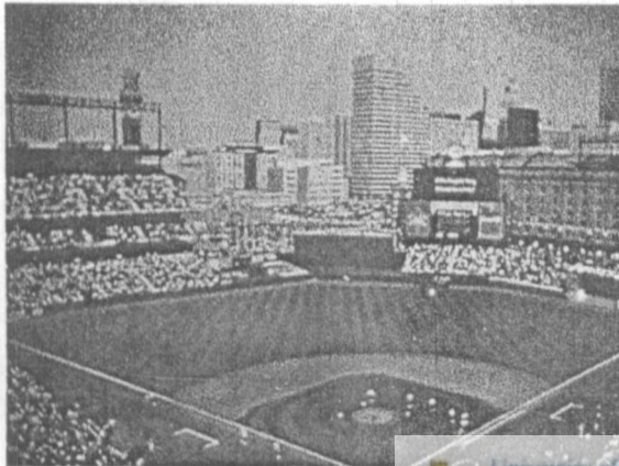
Fig. 3.6.8 Oriole Baseball Park in Camden Yards, USA. 1992. Capacity 48,000
