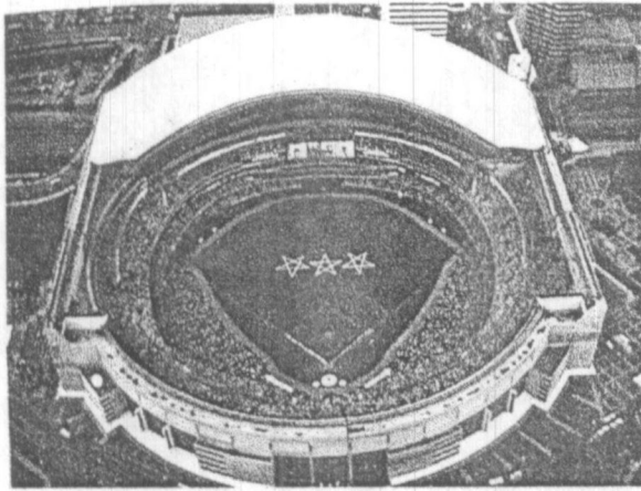
Fig. 2.3.8 Toronto Skydome at Toronto, Canada.
