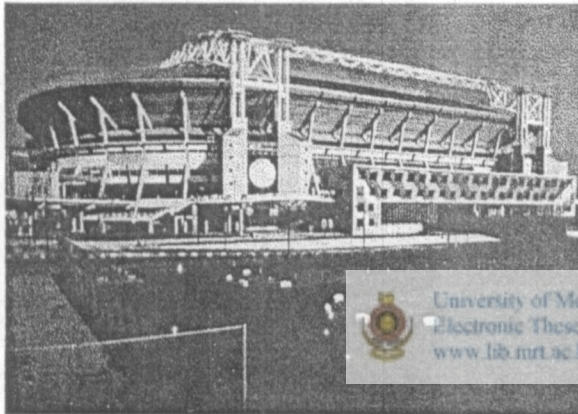
Fig. 2.0.3 Amsterdam Arena at Amsterdam, Netherlands. 1993- 1996
