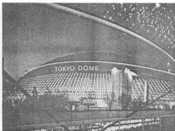
Fig. 3.6.4 Tokyo Dome in Tokyo, Japan. 1985- 1988. Capacity 55,000
