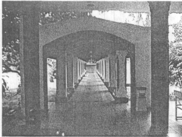
Fig. 4.4.9 Passage between the Entrance Lobby to Restaurant and Ground
