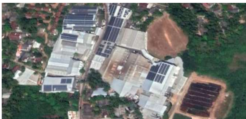
Figure 4.4: Roof-Mounted Grid-Tied PV System of Case D
