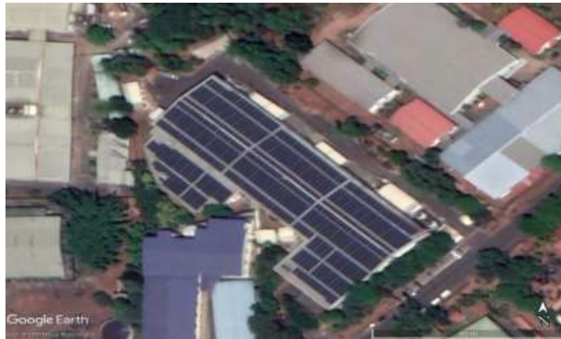
Figure 4.2: Roof-Mounted Grid-Tied PV System of Case B
