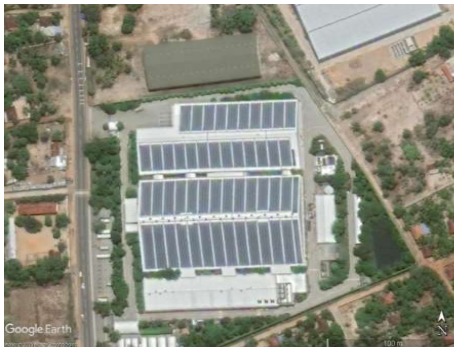
Figure 4.3: Roof-Mounted Grid-Tied PV System at Case C
