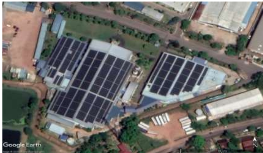
Figure 4.1: Roof-Mounted Grid-Tied PV System at Case A
