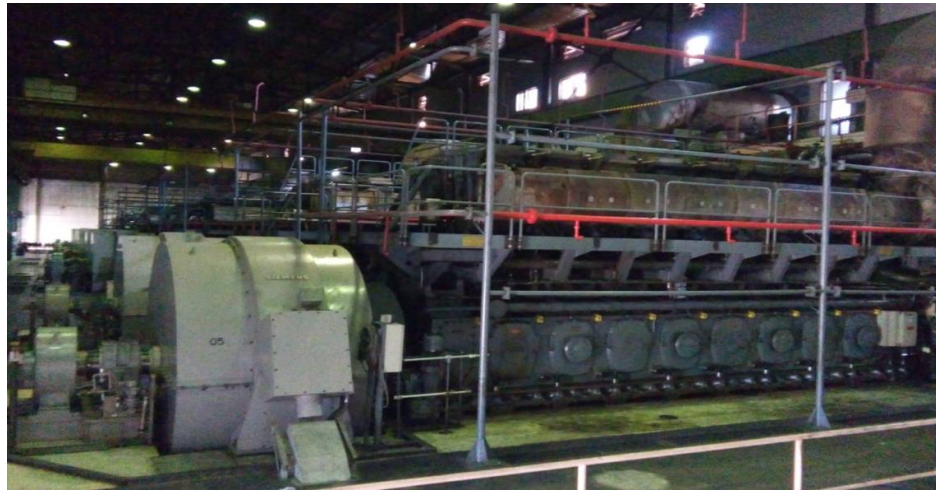
Figure 5:12 Layout of MAN plant Genset
