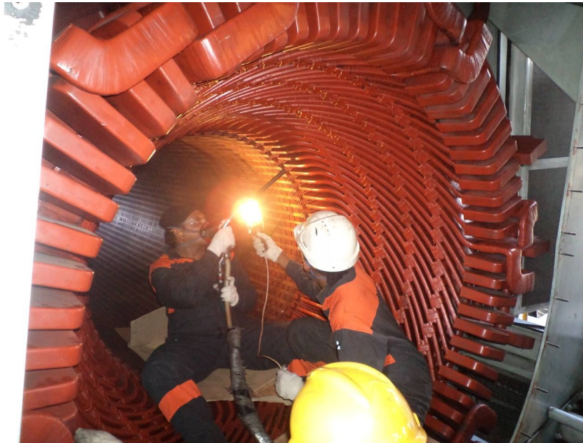
Figure 5:21 Dry ice cleaning work of KPSGT7 during 96,000 Rhr maintenance
