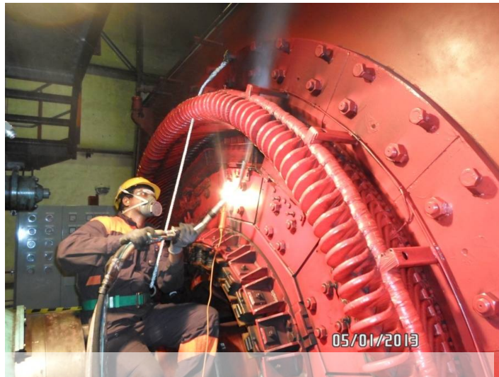
Figure 5:3 Dry Ice cleaning of G4, Sapugaskanda Power Station
