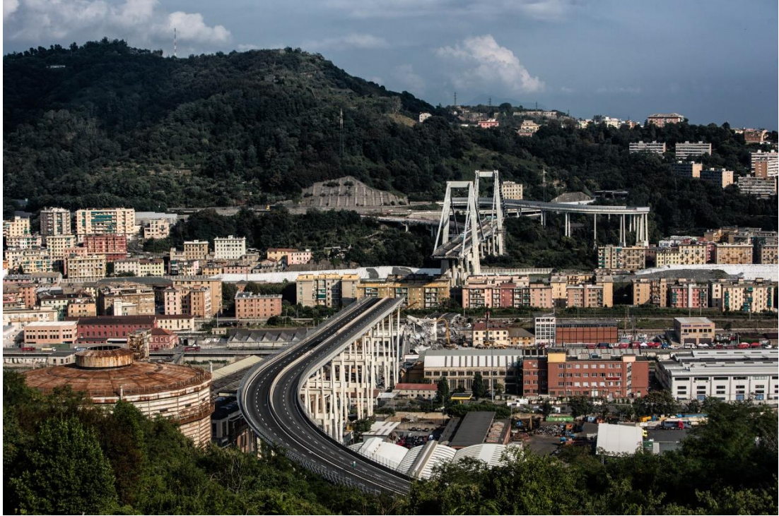
Fig. 2.1: Morandi Bridge collapse [8]
