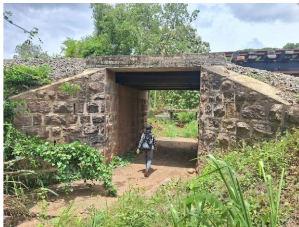
Figure 6: Existing underpass tunnel
