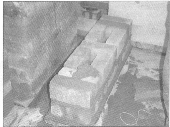
Figure 2 - Rat-trap bond under construction
