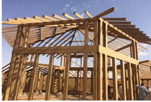
Figure 2.5: Engineered bamboo construction (Wei, 2019(b))
