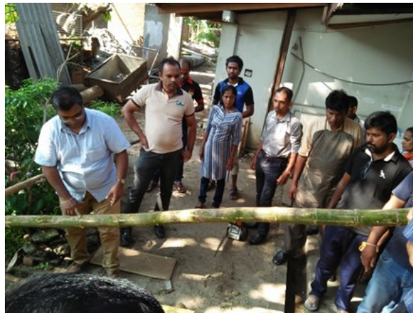
Figure 2.6: Checking straightness of pole
