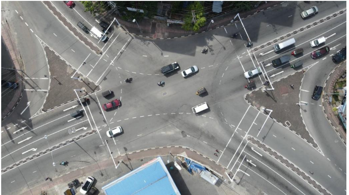
Figure 7 Pelawatta Junction, Pelawatta.-Drone View
