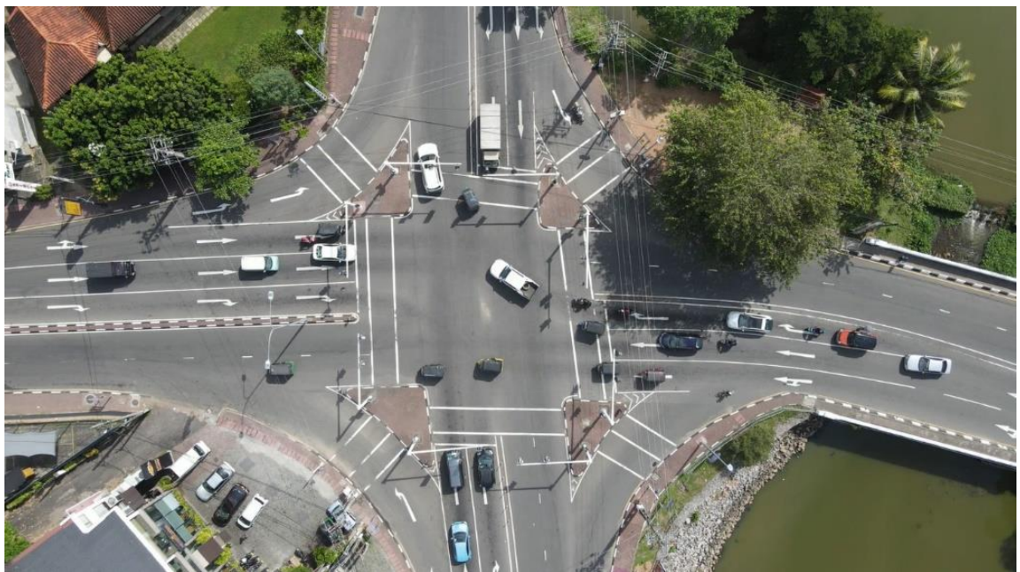
Figure 2 Palamthuna Junction - Drone View
