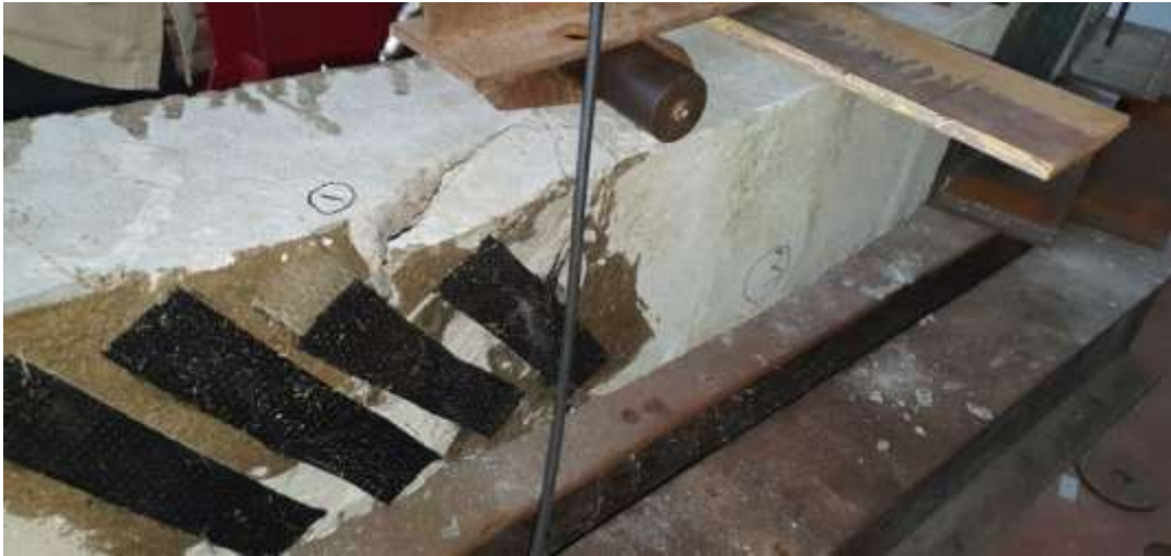
Figure 36: De-bonding of fibre strip and spalling of concrete – Beam
