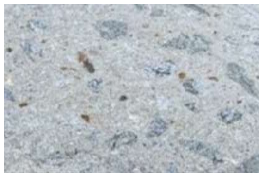
Figure 15: Smoothened substrate after grinding
