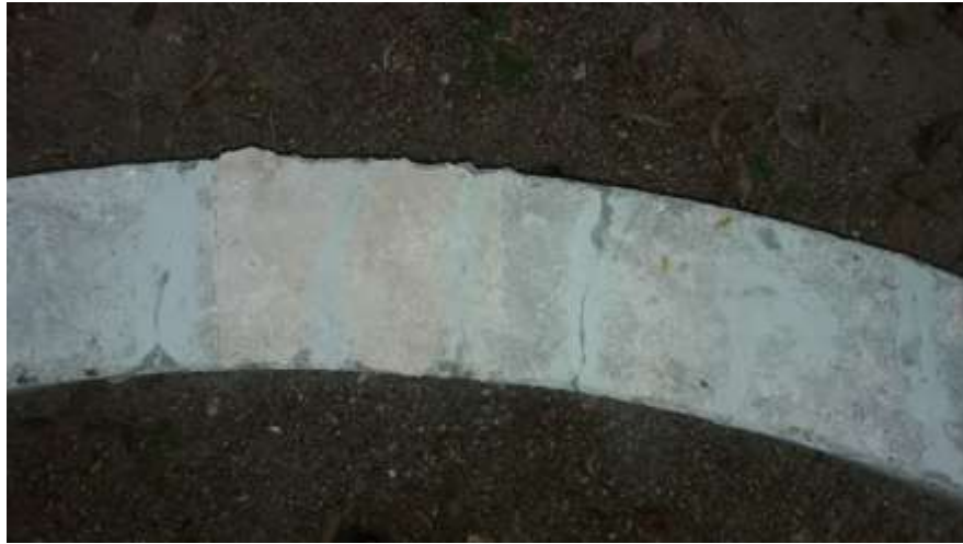
Figure 14: Flexural cracks repaired in beam
