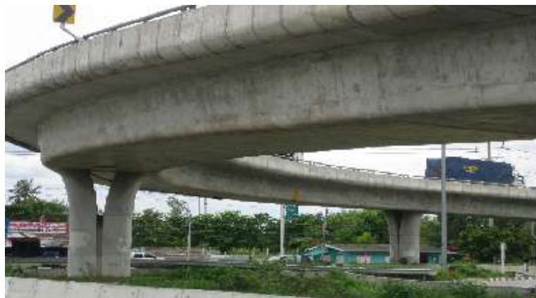
Figure 2: Curved bridge (Yindeesuk, 2009)
