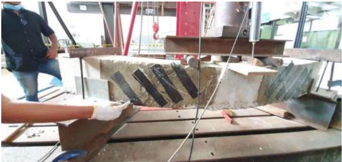
Figure 31: Developing shear cracks – Beam B
