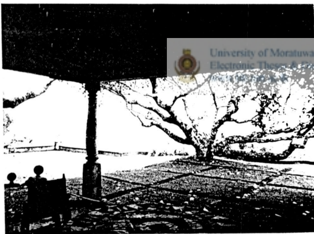
(Figure 66: Limited Penetration by Overhanging roof)
