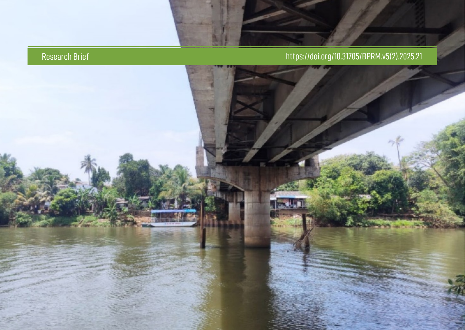
Figure 1: View of the Kelanisiri Bridge across the Kelani River
