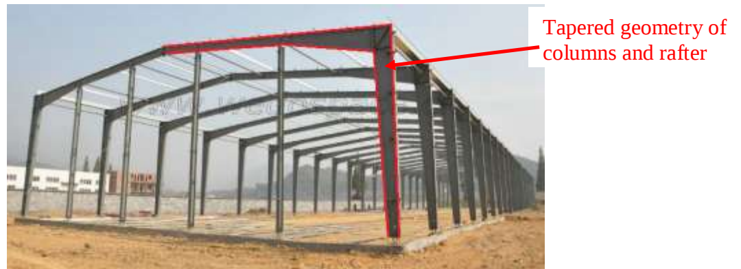
Figure 2.1 Bespoke members shape restricts the reuse on different applications
